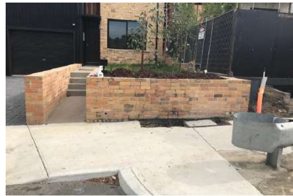
Wall after graffiti removal
